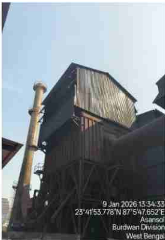
Bag Filter attached with Product house for DRI
