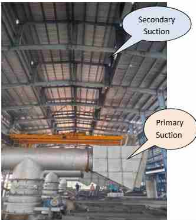
Primary & secondary suction connected with induction
