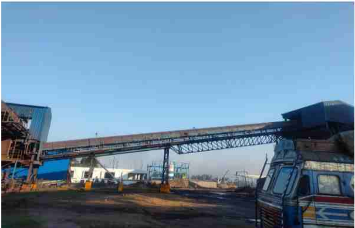
Covered raw material handling
