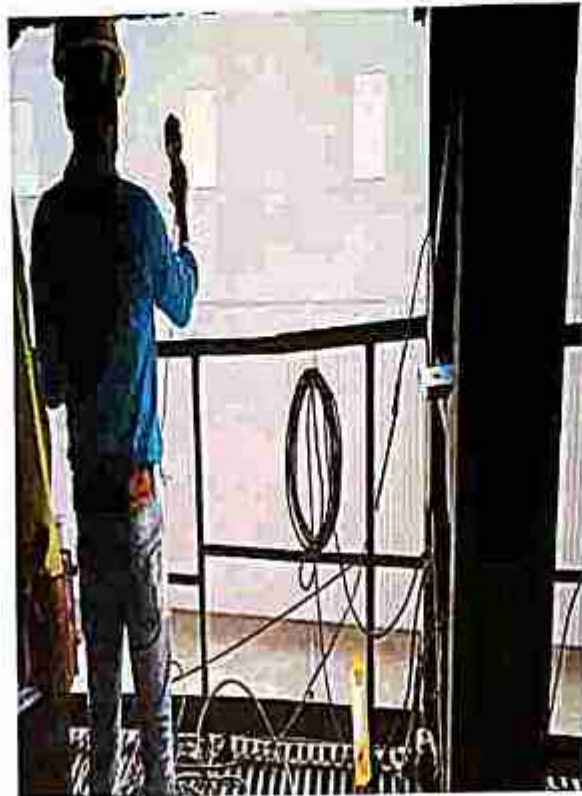
DRI KILN PLATFORM NO - 1 (QRT AREA)
