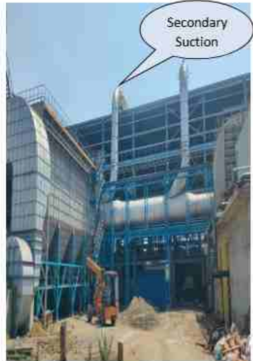
Primary & secondary suction connected with induction
