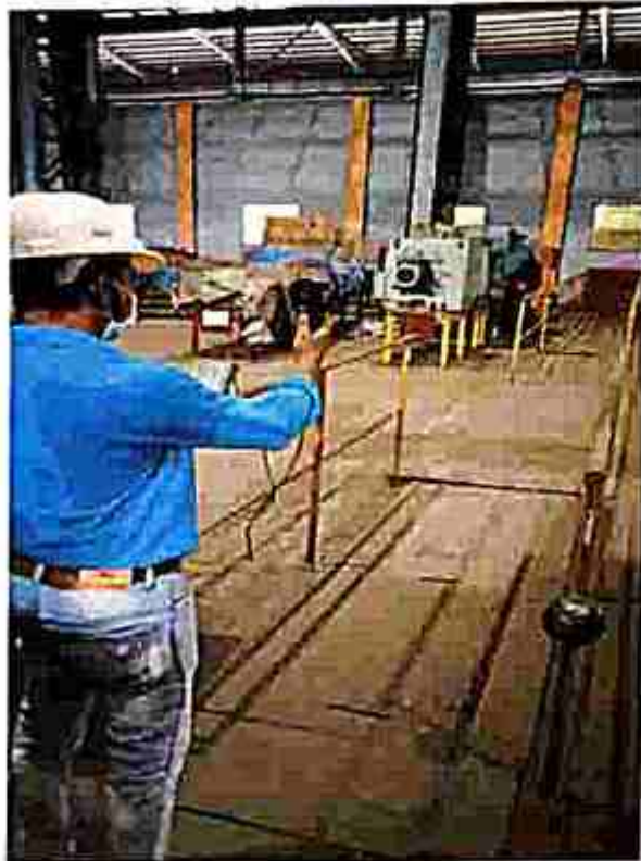
ROLLING MILL BILLET CHAIN TRANSFER AREA
