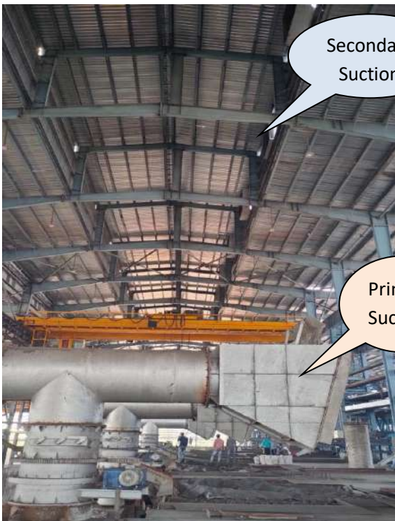
Primary & secondary suction connected with induction
