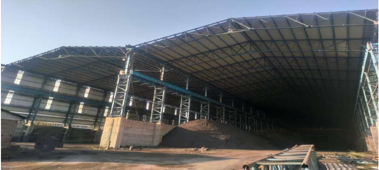
Raw material storage shed
