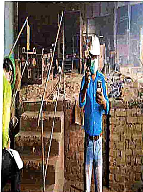
FERRO TAPING AREA
