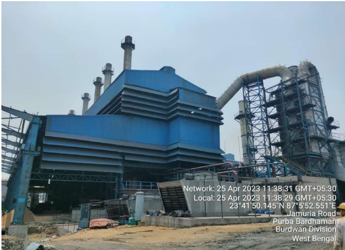
Bag Filter connected with 2x9 MVA SEAF
