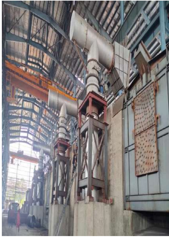
Bag Filter for Steel Smelting Shop
