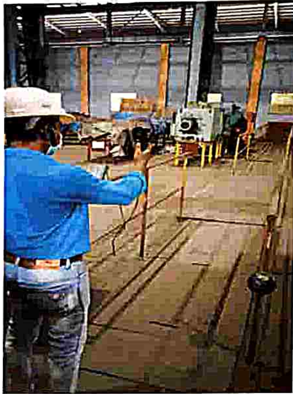
ROLLING MILL BILLET CHAIN TRANSFER AREA
