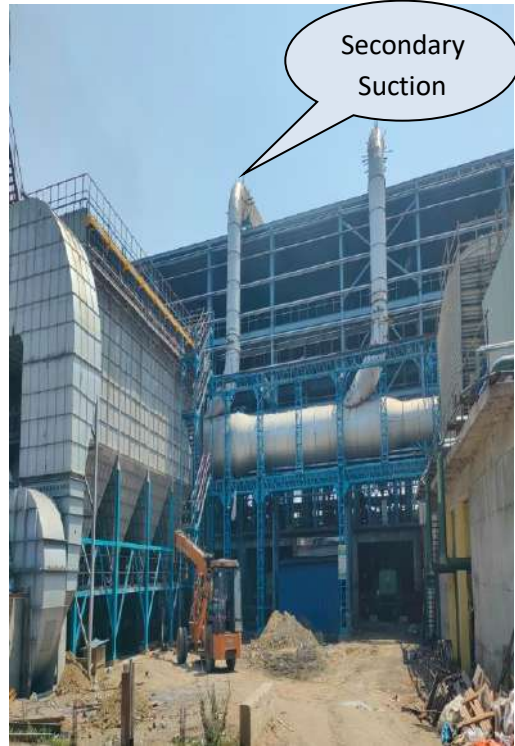
Primary & secondary suction connected with induction
