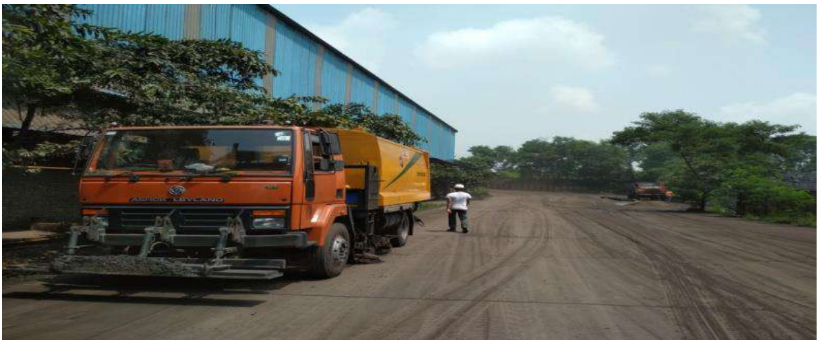
Road sweeping machine to control fugitive dust from road during transportation
