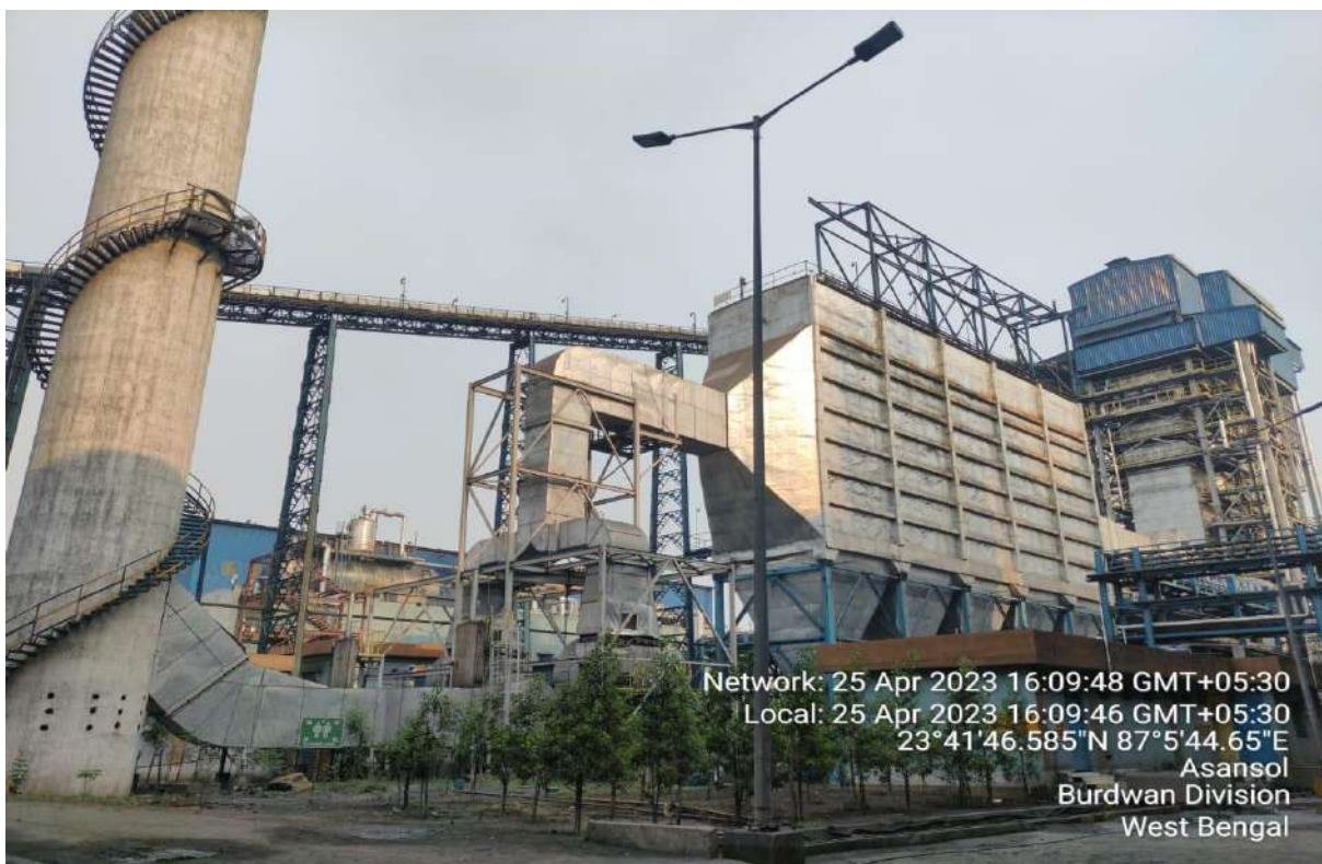
5 field ESP for CFBC Boiler
