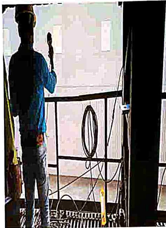
DRI KILN PLATFORM NO - 1 (QRT AREA)
