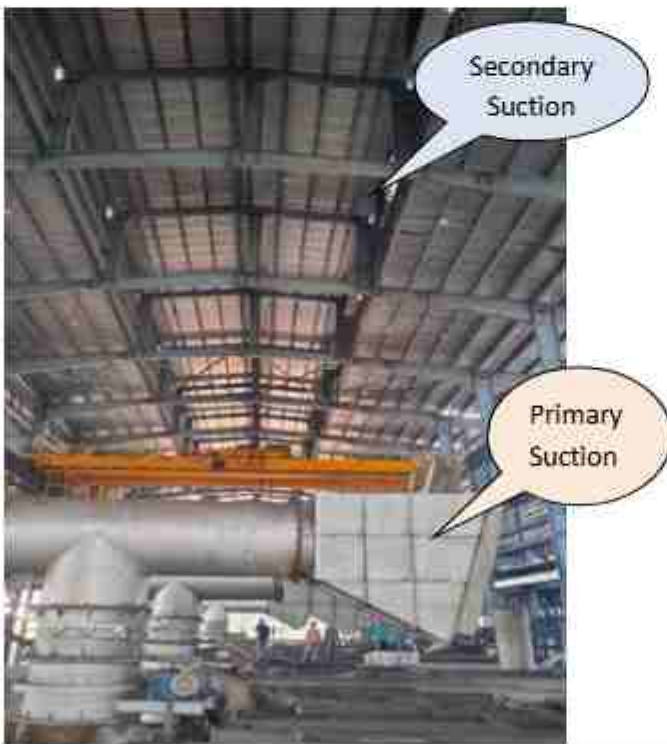
Primary & secondary suction connected with induction
