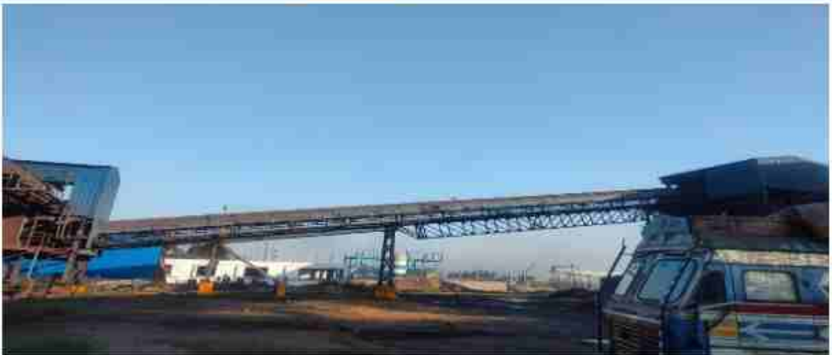
Closed Conveyor for raw materials handling
