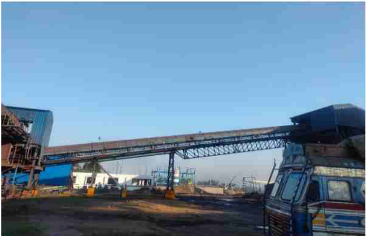
Covered raw material handling
