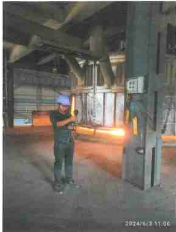
FERRO FURNACE FLOOR
