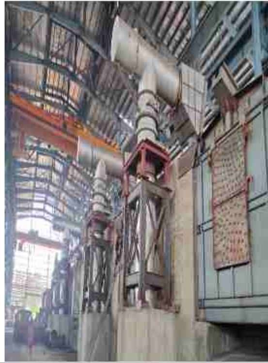
Induction furnace connected with primary hood
