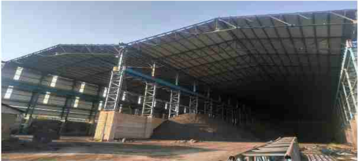
Raw material storage shed
