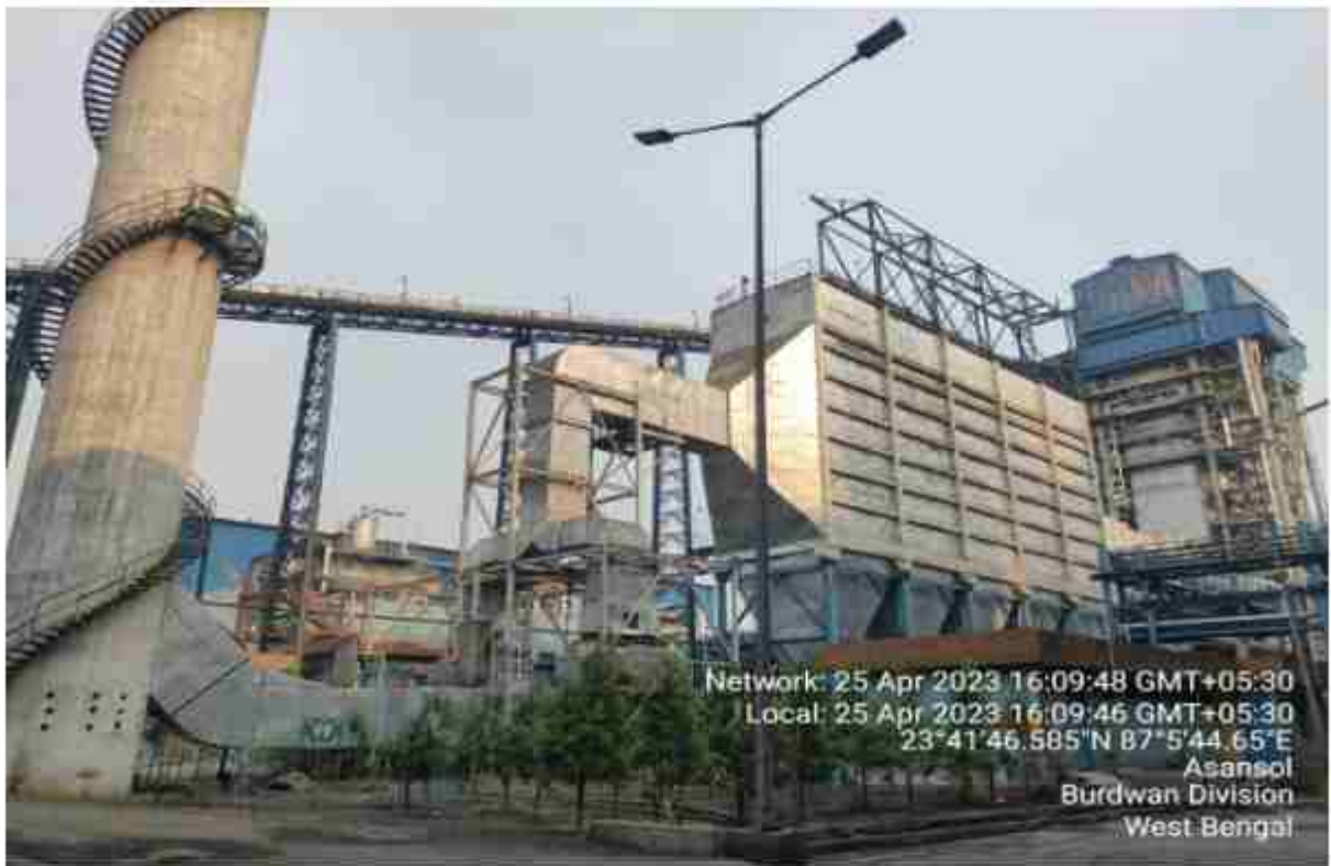
5 field ESP for CFBC Boiler
