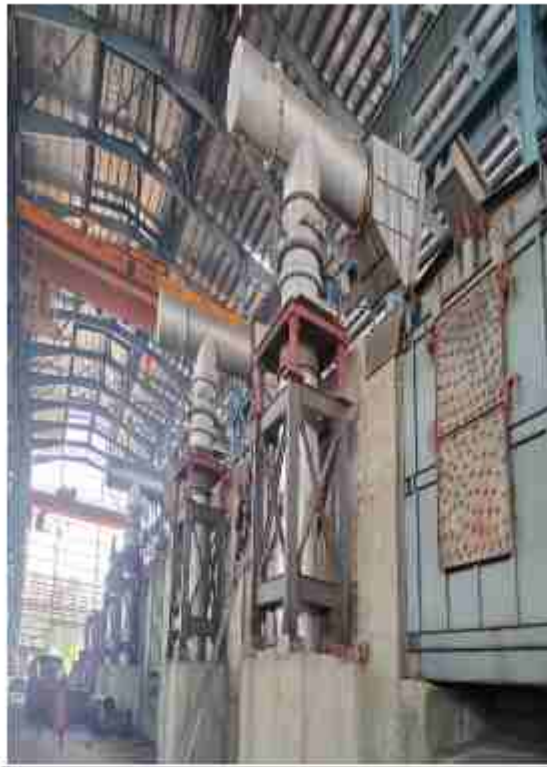
Bag Filter for Steel Smelting Shop
