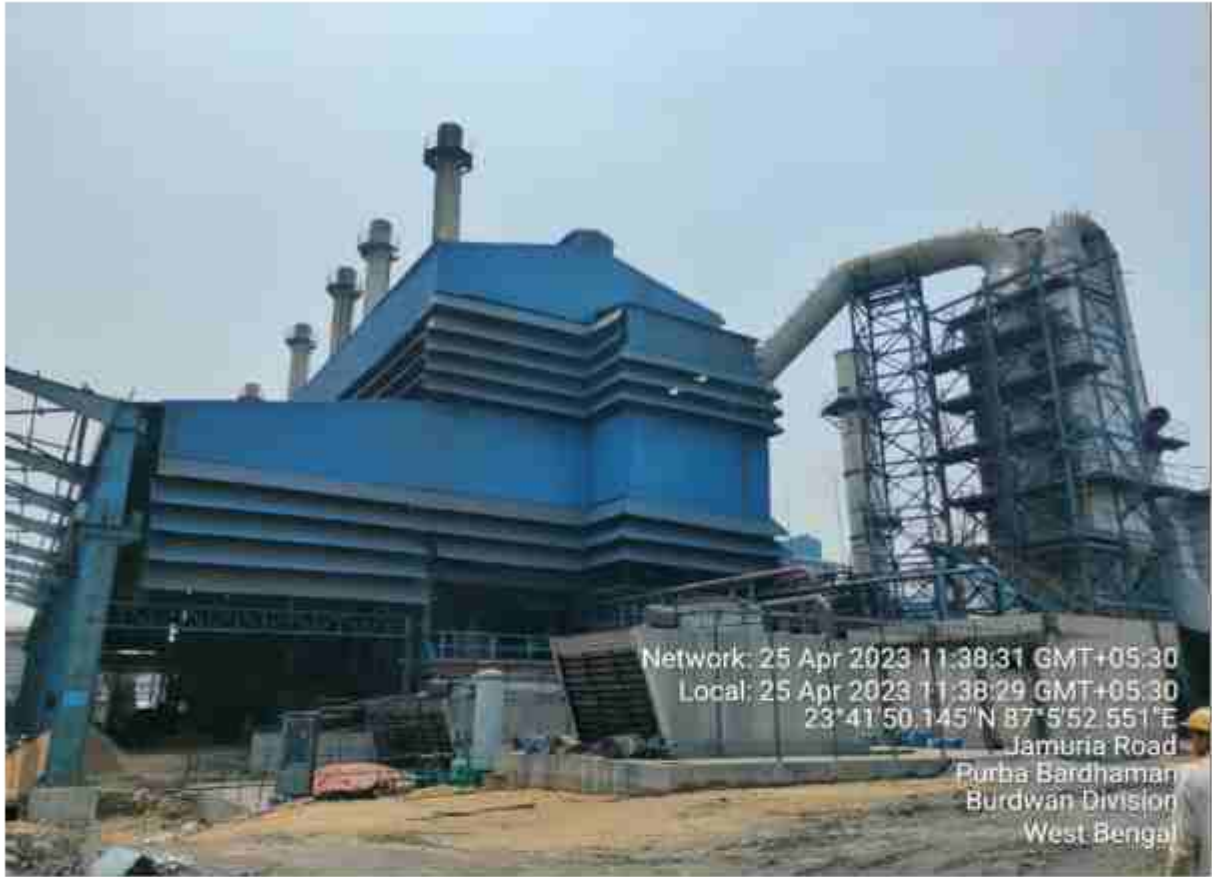
Bag Filter connected with 2x9 MVA SEAF
