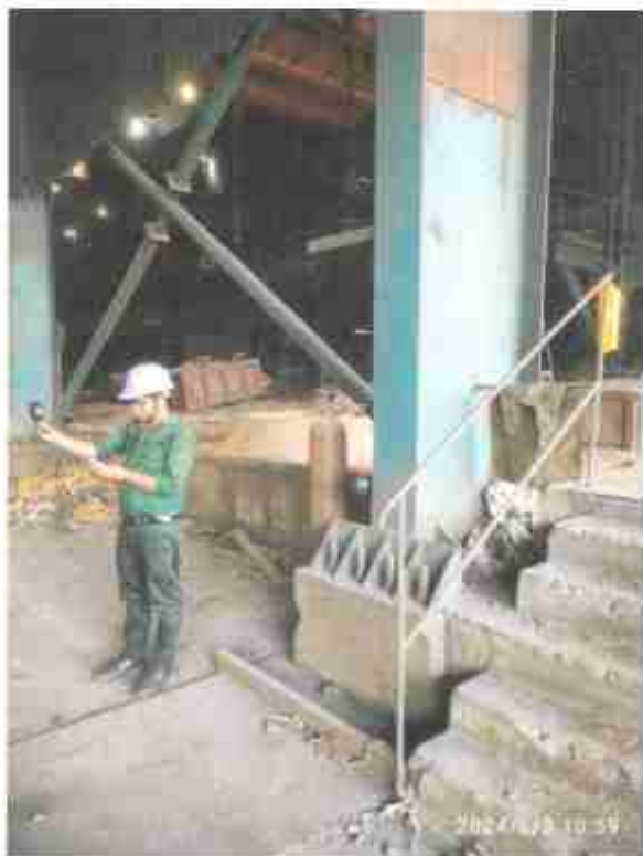
FERRO TAPING AREA
