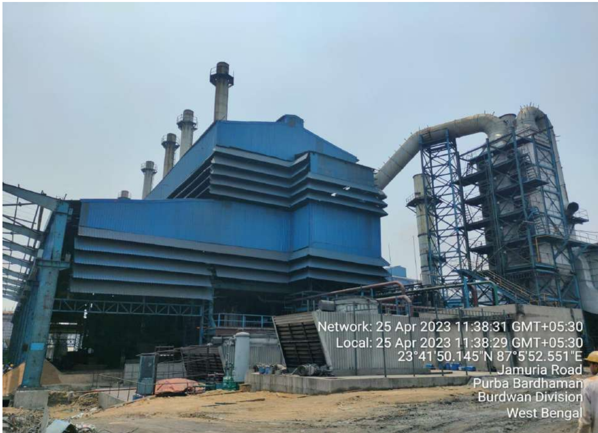
Bag Filter connected with 2x9 MVA SEAF
