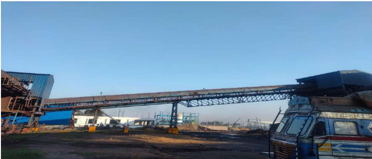
Closed Conveyor for raw materials handling
