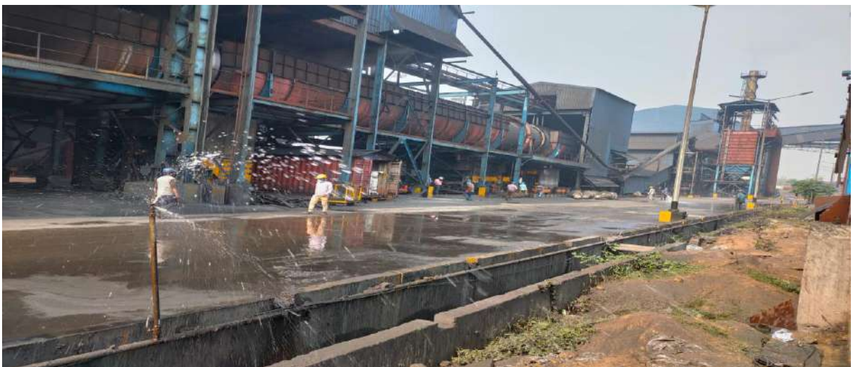
Water Sprinkler on road of plant site
