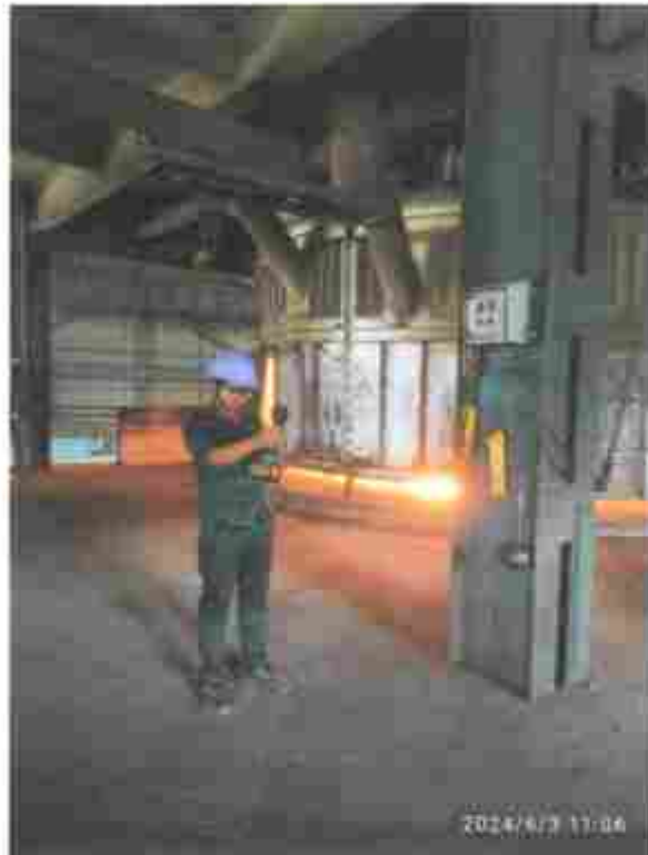
FERRO FURNACE FLOOR
