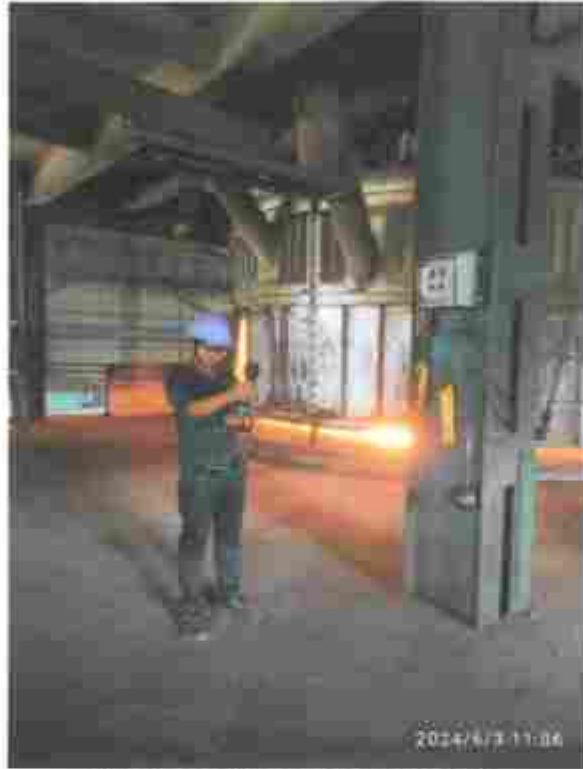
FERRO FURNACE FLOOR
