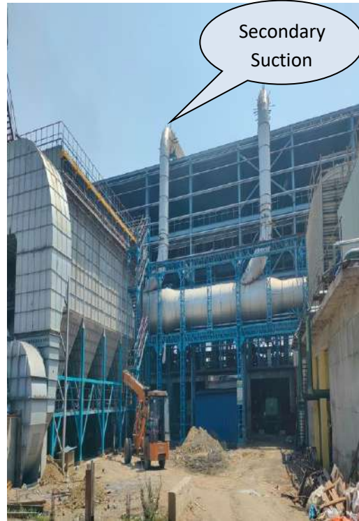
Primary & secondary suction connected with induction
