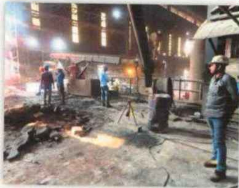
FURNACE PLATFORM NEAR FURNACE NO - 03
