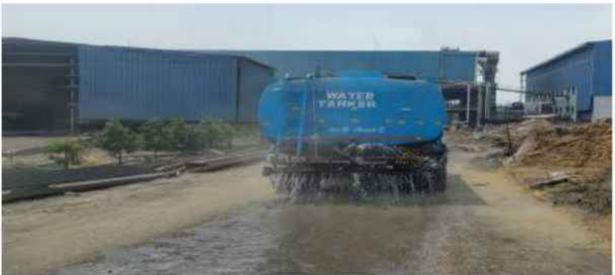
Water tanker for sprinkling on road of project site
