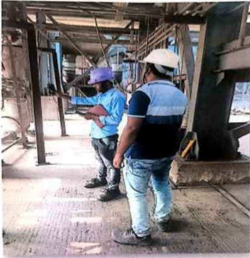
CPP WHRB BOILER NO - 02
