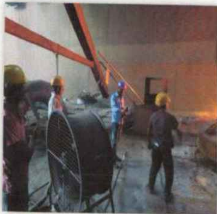
FURNACE PLATFORM NEAR FURNACE NO. - 01
