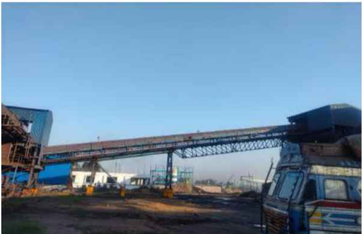
Covered raw material handling
