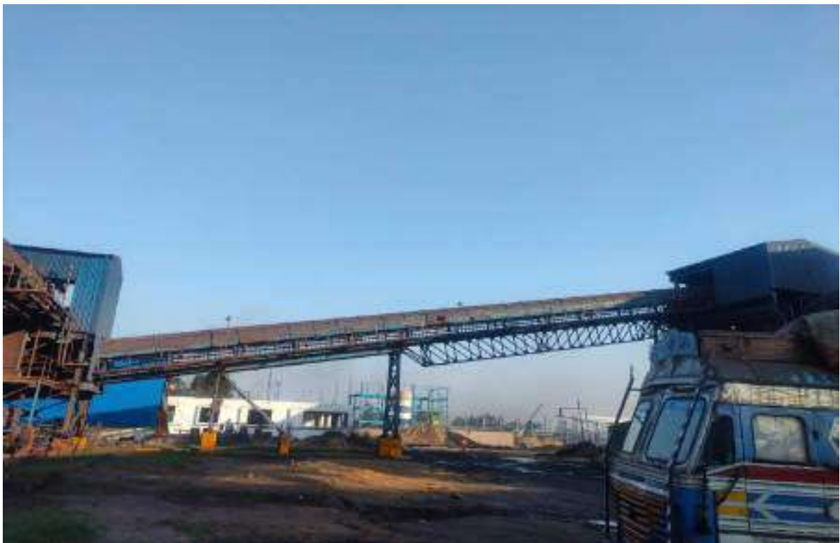
Covered raw material handling
