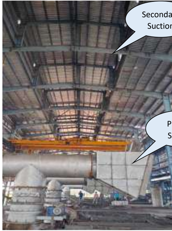
Bag Filter for Steel Smelting Shop
