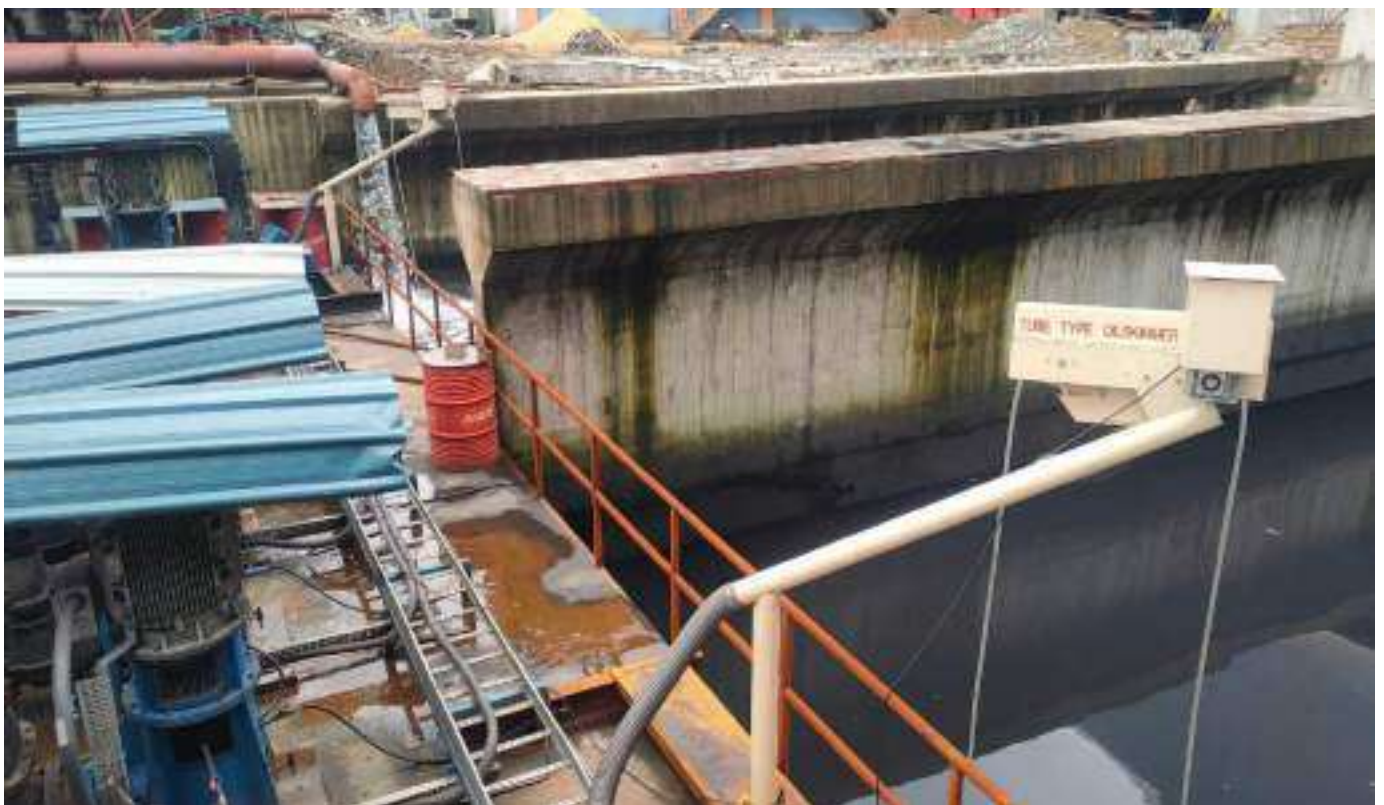
Oil Skimmer for Oil Removal
