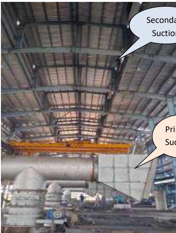
Primary & secondary suction connected with induction
