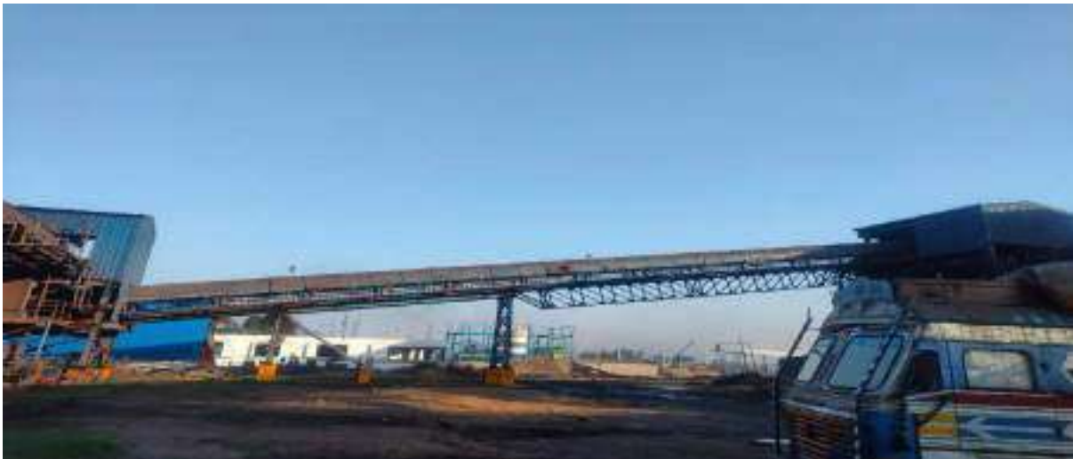
Closed Conveyor for raw materials handling
