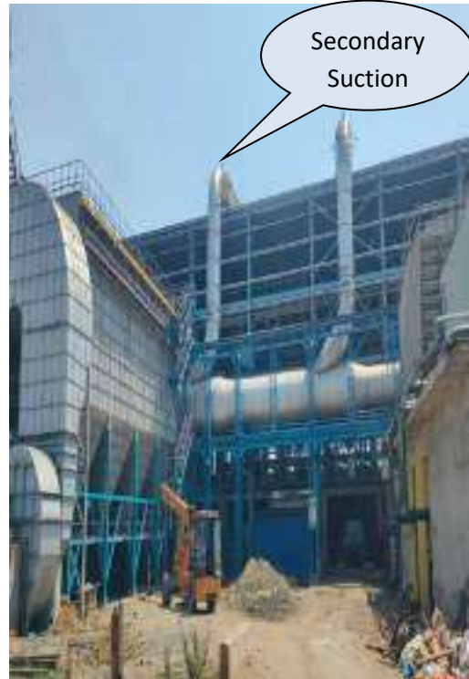
Primary & secondary suction connected with induction
