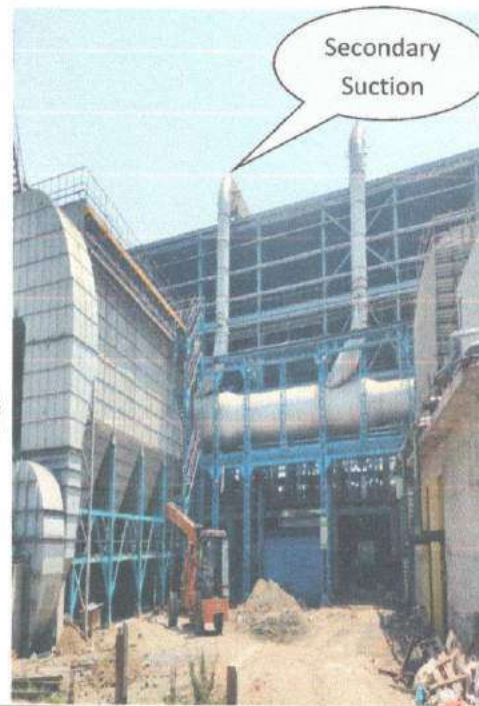
Primary & secondary suction connected with induction
