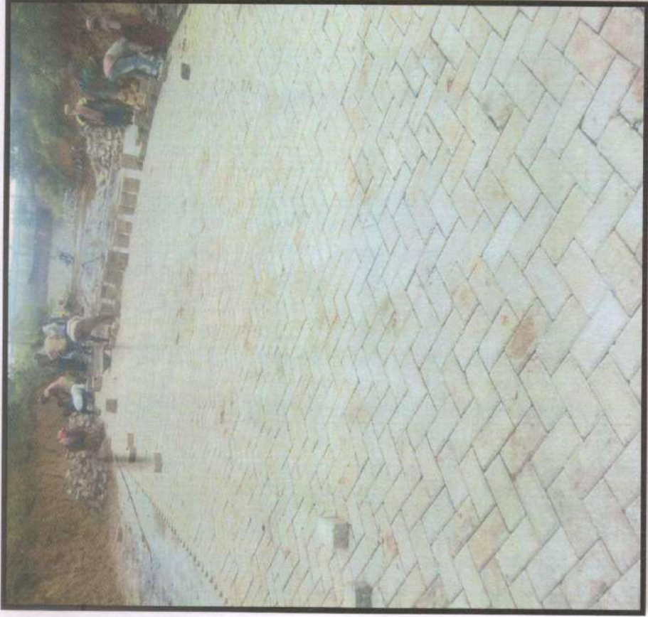
Damodarpur More adjacent to Jamuria Haripur main road repairing work by heavy duty paver blocks
