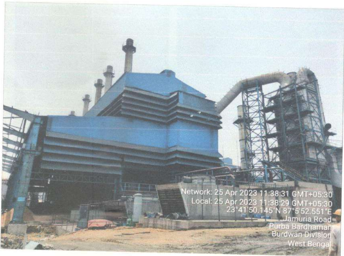
Bag Filter connected with 2x9 MVA SEAF
