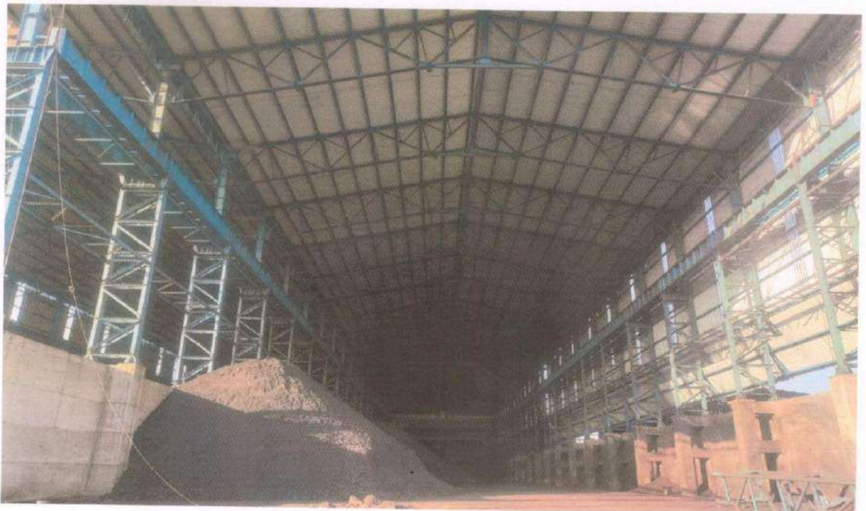
Raw material stock yard
