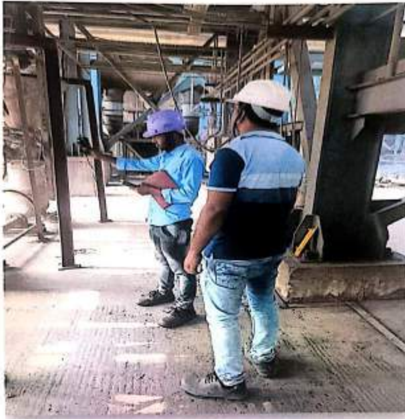
CPP WHRB BOILER NO - 02
