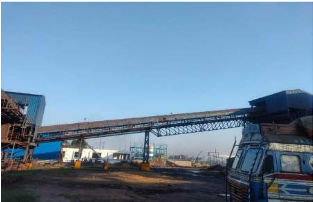
Covered raw material handling
