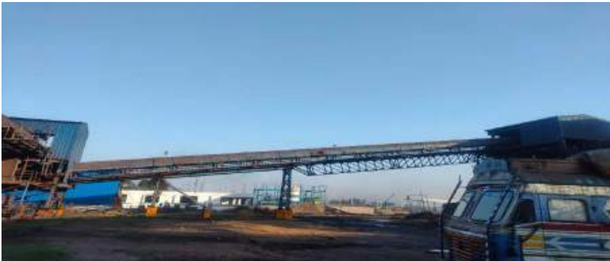
Closed Conveyor for raw materials handling
