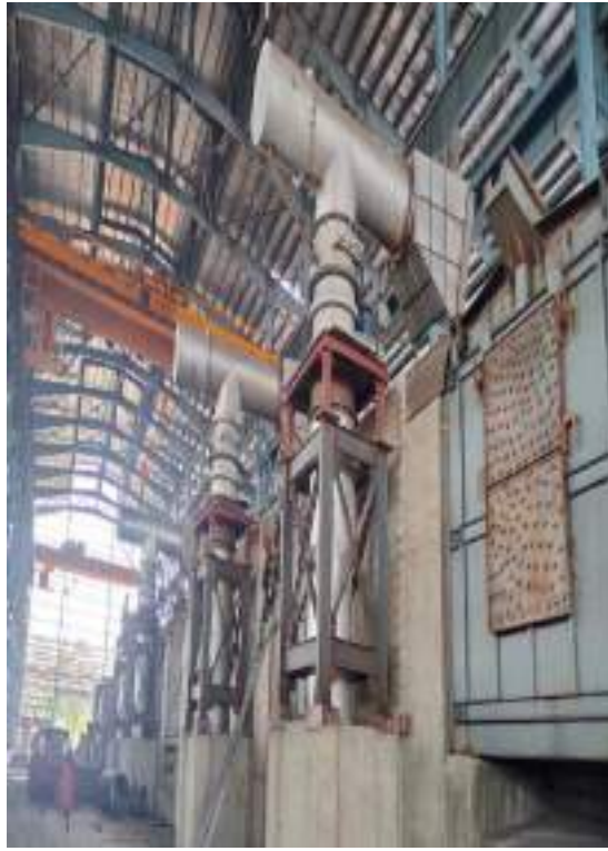
Bag Filter for Steel Smelting Shop
