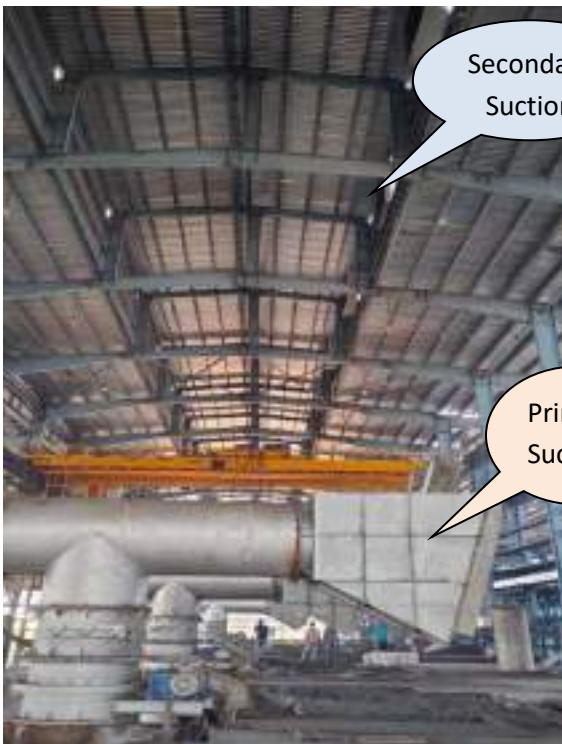
Primary & secondary suction connected with induction
