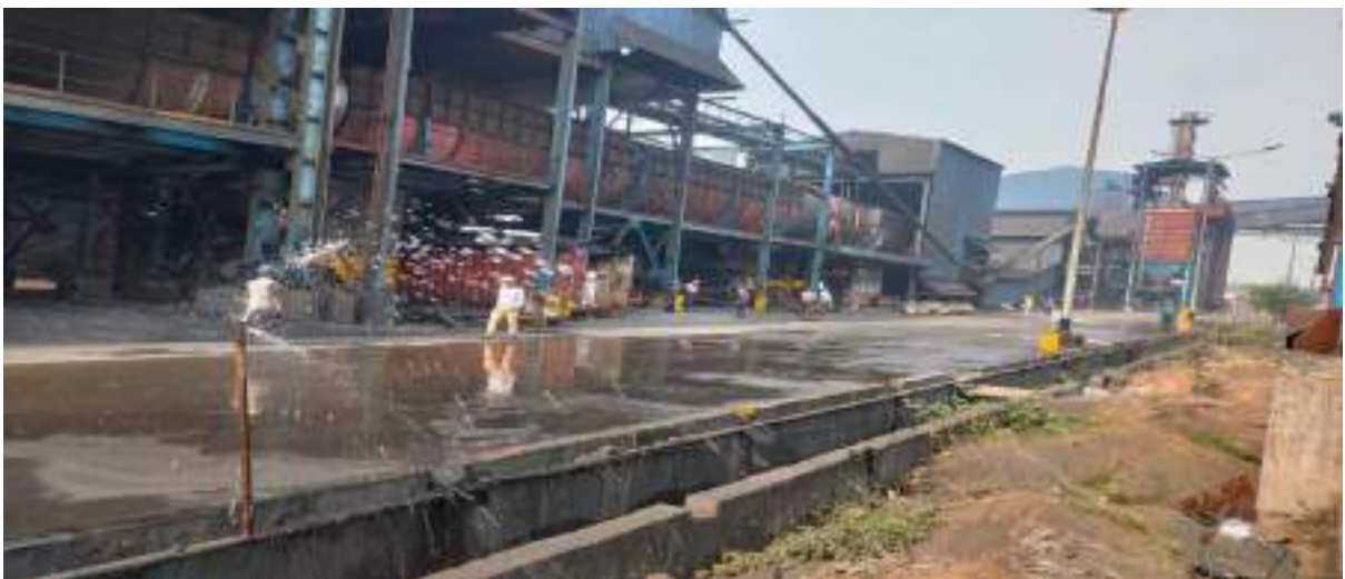
Water Sprinkler on road of plant site
