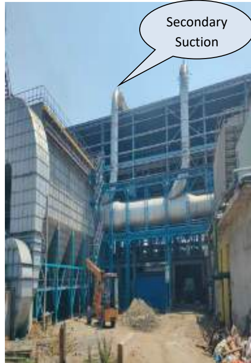
Primary & secondary suction connected with induction
