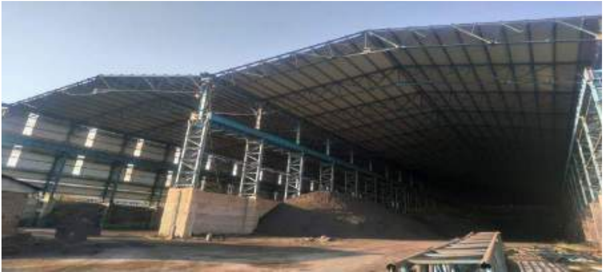
Raw material storage shed
